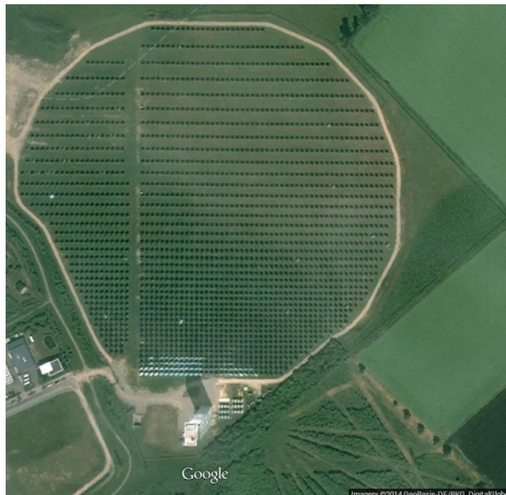
Figure 13: Heliostat field of Jülich plant, Germany
