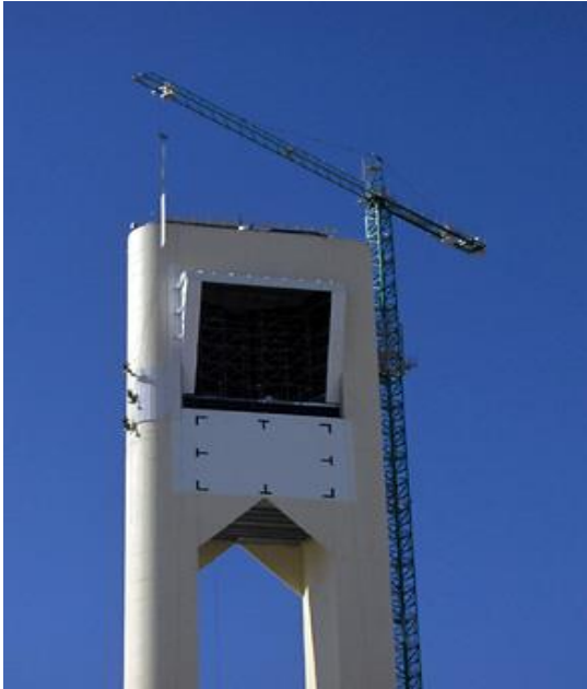
Figure 3: Cavity Receiver used in PS-10
