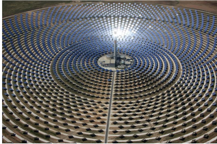
Figure 1: Gemastar Power Plant
